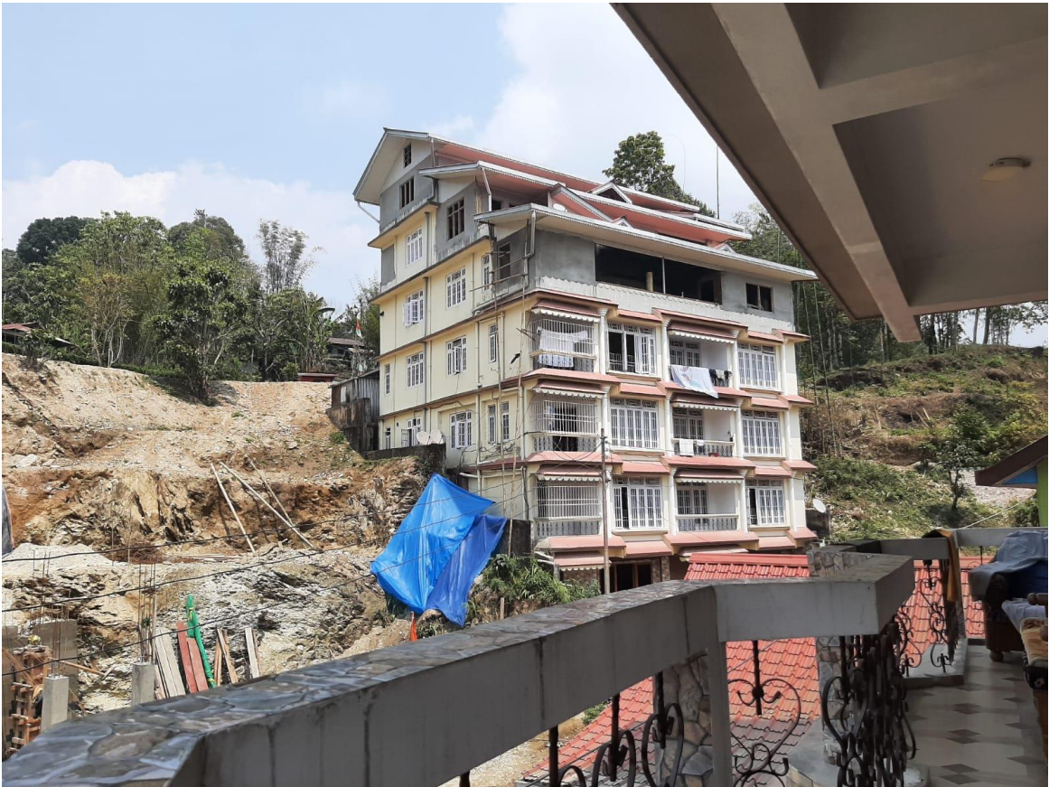
Plate 3: Construction of new hotels on the hillslope of Aritar, Eastern Sikkim
