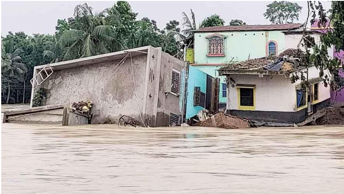
Figure 9: A two-storey house, which went under water at the flooded-Bandar village near Khanakul in Hooghly district three days ago, completely collapsed on early Tuesday morning. Source: P.C.: Ananda Adhikari; https://www.telegraphindia.com/west-bengal/building-crumbles-at-the-flooded-bandar-village-near-khanakul-in-hooghly/cid/1825197 accessed on 25th June 2023)
